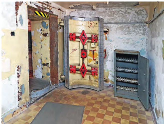
The outer 2.5 tonne blast door added by the Soviets, with curved embrasure. Photo Clive Penfold
